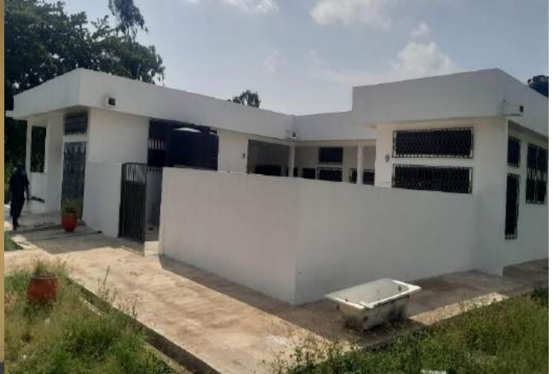
REFURBISHMENT OF DCE'S RESIDENCE
