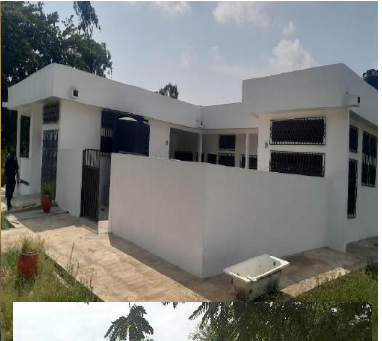
REFURBISHMENT OF DCE'S RESIDENCE
