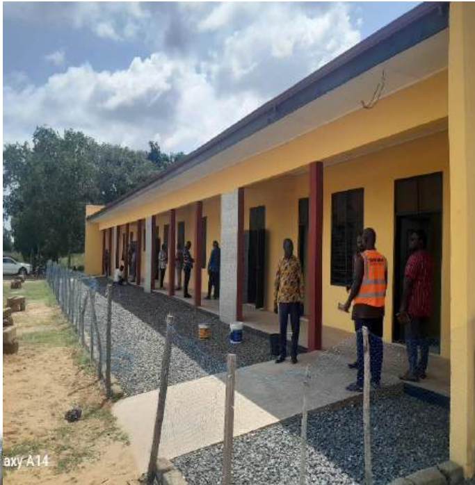
CONSTRUCTION OF 3-UNIT CLASSROOM BLOCK AT
