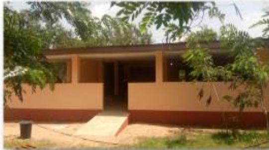
CONSTRUCTED OPD AT KPOTAME CHPS COMPOUND
