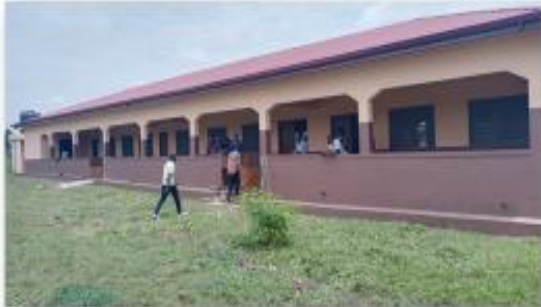
CONSTRUCTED 3-UNIT CLASSROOM BLOCK WITH 2-SEATER WC TOILET FOR ICCESS AT SOGAKOPE
